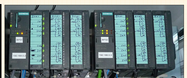
Top: Hardware installation of the PLC system containing two sets of: PLC satellite controller, relay module, DAC module (2x).
