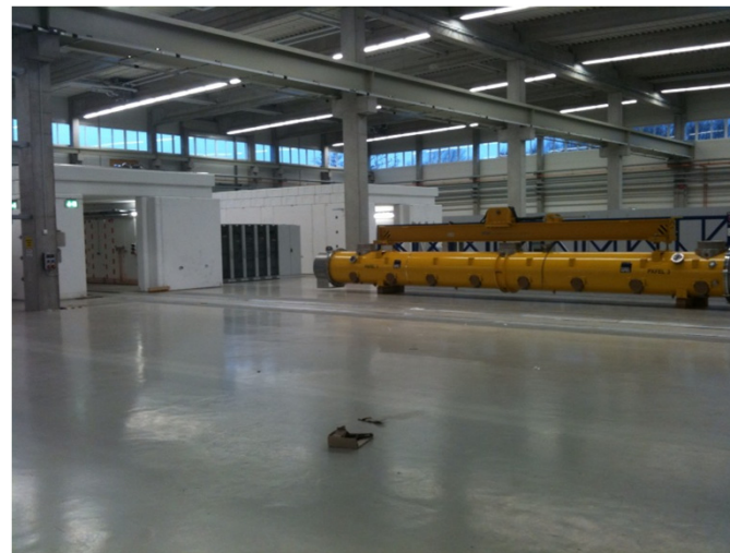
Feb 2011: Test stands under construction
