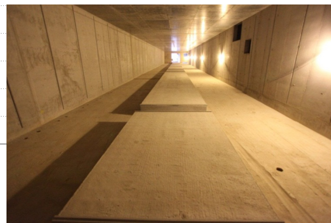
Level 7 of injector building
