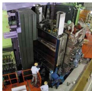
Figure 3: Photo of installing the accelerating cavity(RES2) and the flattopping(FT) cavity to the valley area between the sector #2 and #3.
