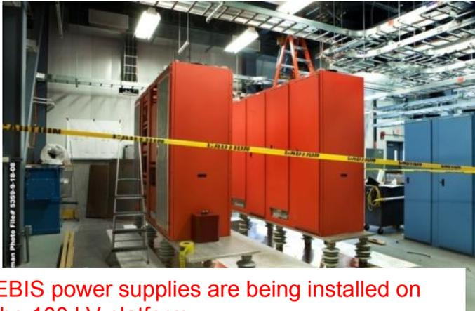
EBIS power supplies are being installed on the 100 kV platform
