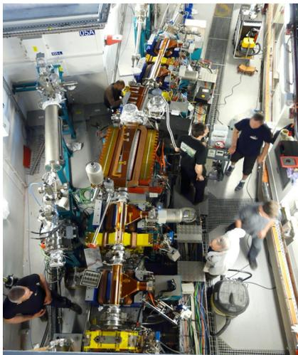
Figure 3: Installation of the new dipole vacuum chamber and first diagnostics.
