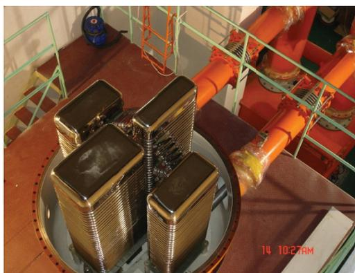
Figure 3: The 1.2 MV/50 mA power supply.
