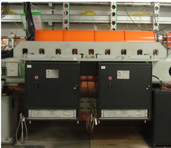
Figure 3: Extraction kicker pulsers installed in the booster extraction straight.
