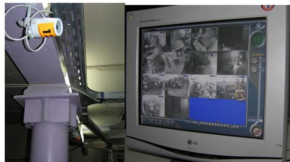
Figure 6: Elements of video monitoring system.
