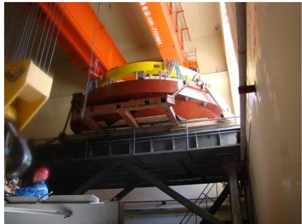
Figure 5: The magnet part on the bracket.
