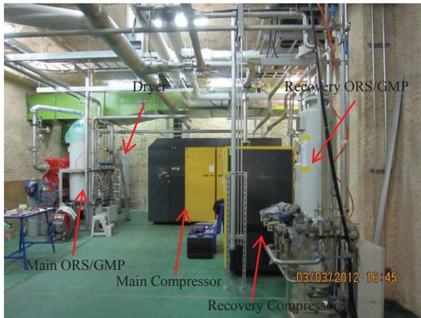
Figure 2a: Layout of the compressor area.
