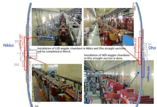
Figure 6: Wiggler magnets and antechamber-type beam pipes installed in the Nikko and Oho straight sections.
