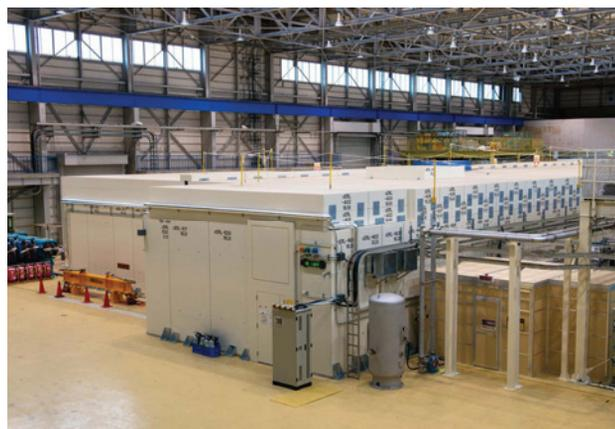
Figure 1: Radiation shielding for the Compact ERL.
