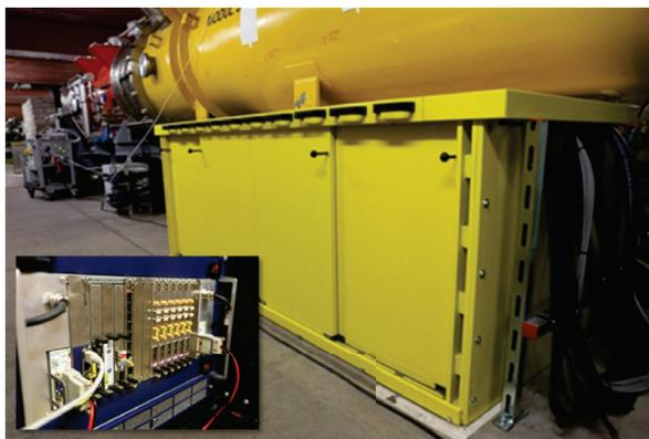
Figure 1: LLRF installation for the first accelerator controls in FLASH underneath the superconducting cryomodule ACC1. Within the small picture an inside view of the rack is given. The yellow housing is a radiation shield protecting internal electronics.
