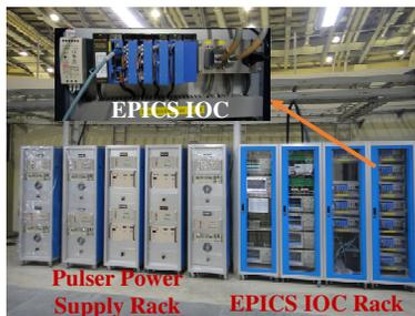
Figure 3: TPS pulse magnets power supplies rack and EPICS IOCs rack.
