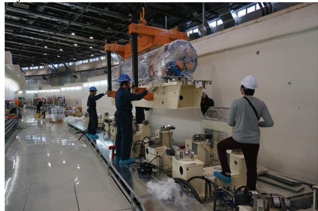
Figure 12: Girder installing with a cradle by a crane.
