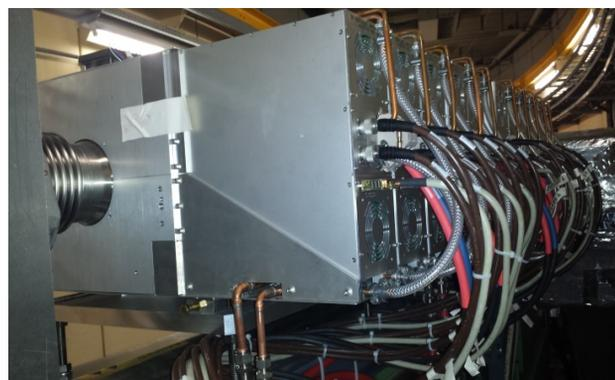
Figure 1: 10-cell prototype MA cavity in PSB Ring 4.
