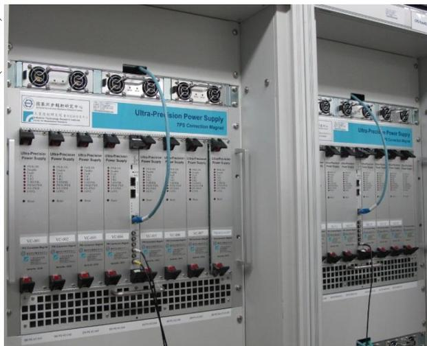
Figure 4: SPS/CPS power converter modules.
