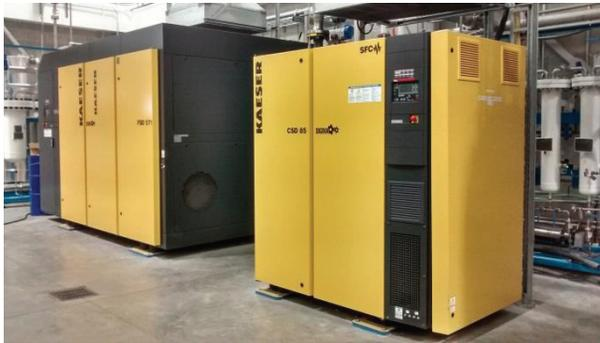
Figure 2: Main and recovery/purification compressors.
