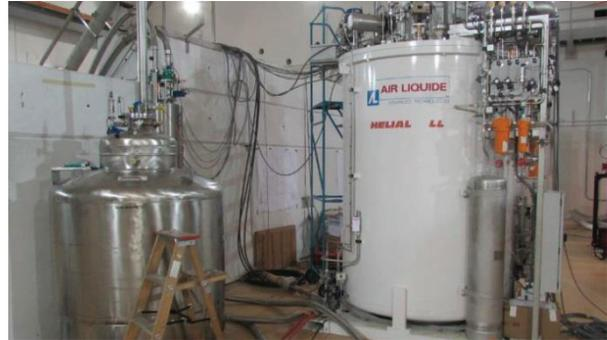
Figure 3: Helium cryoplant during commissioning phase.
