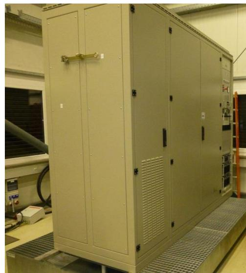
Figure 7: Klystron modulator installed in place.
