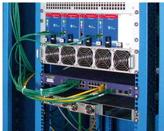
Figure 5: ancillary devices (bottom to top). Bulk AC/DC PS, Ethernet switch, fan unit, A2620 crate.
