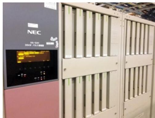
Figure 4: NEC 30 kW amplifier for the Buncher-1 cavity.
