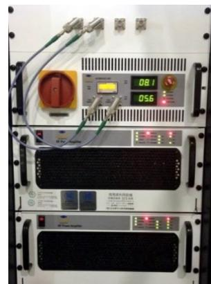
Figure 5: TOMOCO 30 kW amplifier for the Buncher-2 cavity.
