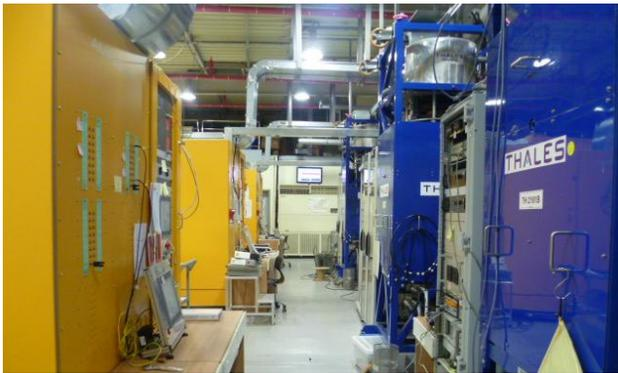
Figure 2: Three 300kW klystrons and KSUs.
