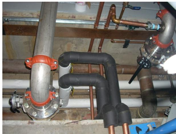
Figure 5: New Chilled Water Lines (insulated pipes in this photo).
