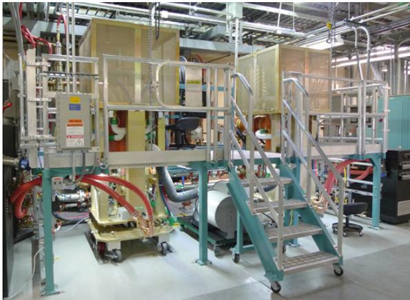
Figure 3: Dual FPAs with Diacrodes<sup>®</sup> installed.
