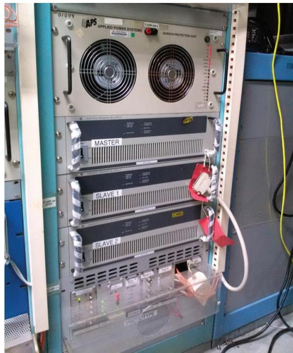
Figure 1: 3 Keeco 10-100GL Units In Parallel.
