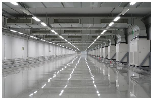
Figure 8: Picture of the 250-m long hard X-ray undulator hall. The ambient temperature control systems are mounted onto the right hand side wall.
