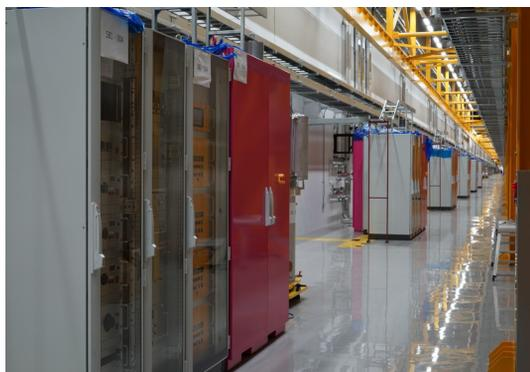
Figure 5: Klystron modulators at the klystron gallery.
