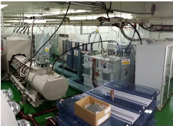
Figure 5: Photo of the 1.2 MW, 324 MHz klystron and its modulator power supply.
