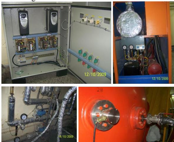
Figure 6: VFD, chiller, piping and connection with tank
