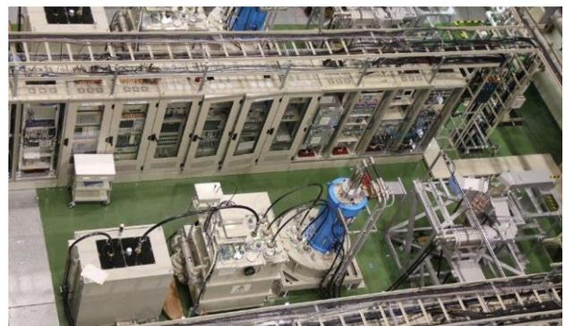
Figure 6: 972 MHz Klystron station. (From left to right) Disconnecting switch, m-anode modulator, klystron tank and circulator. A waveguide is disconnected for maintenance work.
