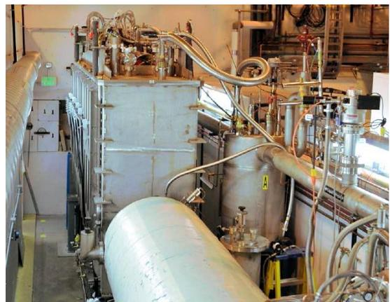
Figure 4: The new Intensity Upgrade cryostat (the rectangular vessel) in the ATLAS tunnel
