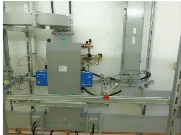
Figure 6: 5 MW power divider and 1 MW isolator in the AMTF shielding tunnel.
