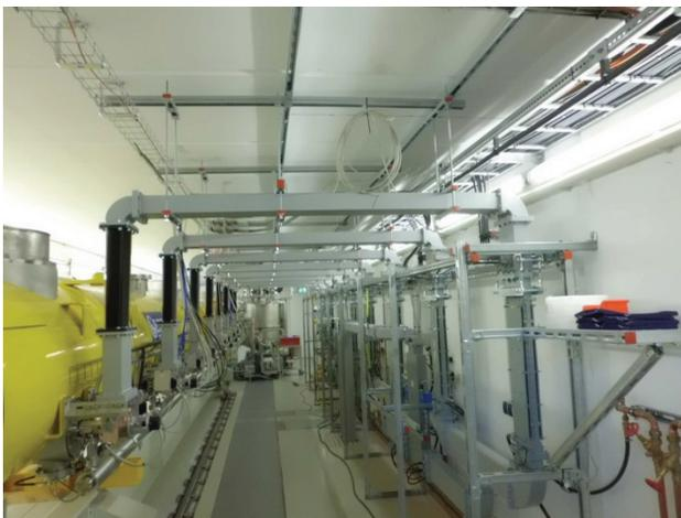
Figure 5: Waveguide distribution connected to a cryomodule in the AMTF shielding tunnel.
