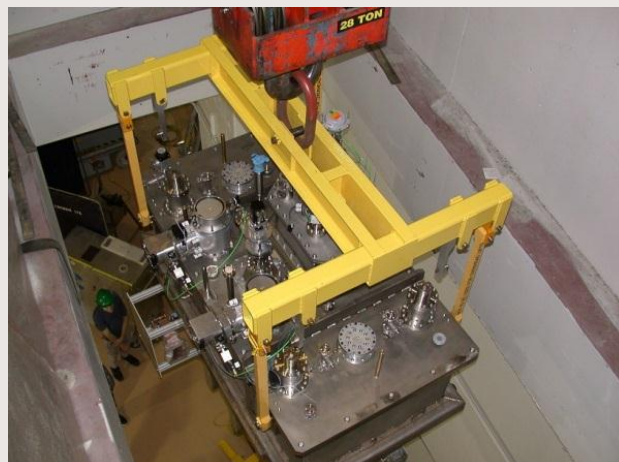
Lowering ICM to the e-Hall
