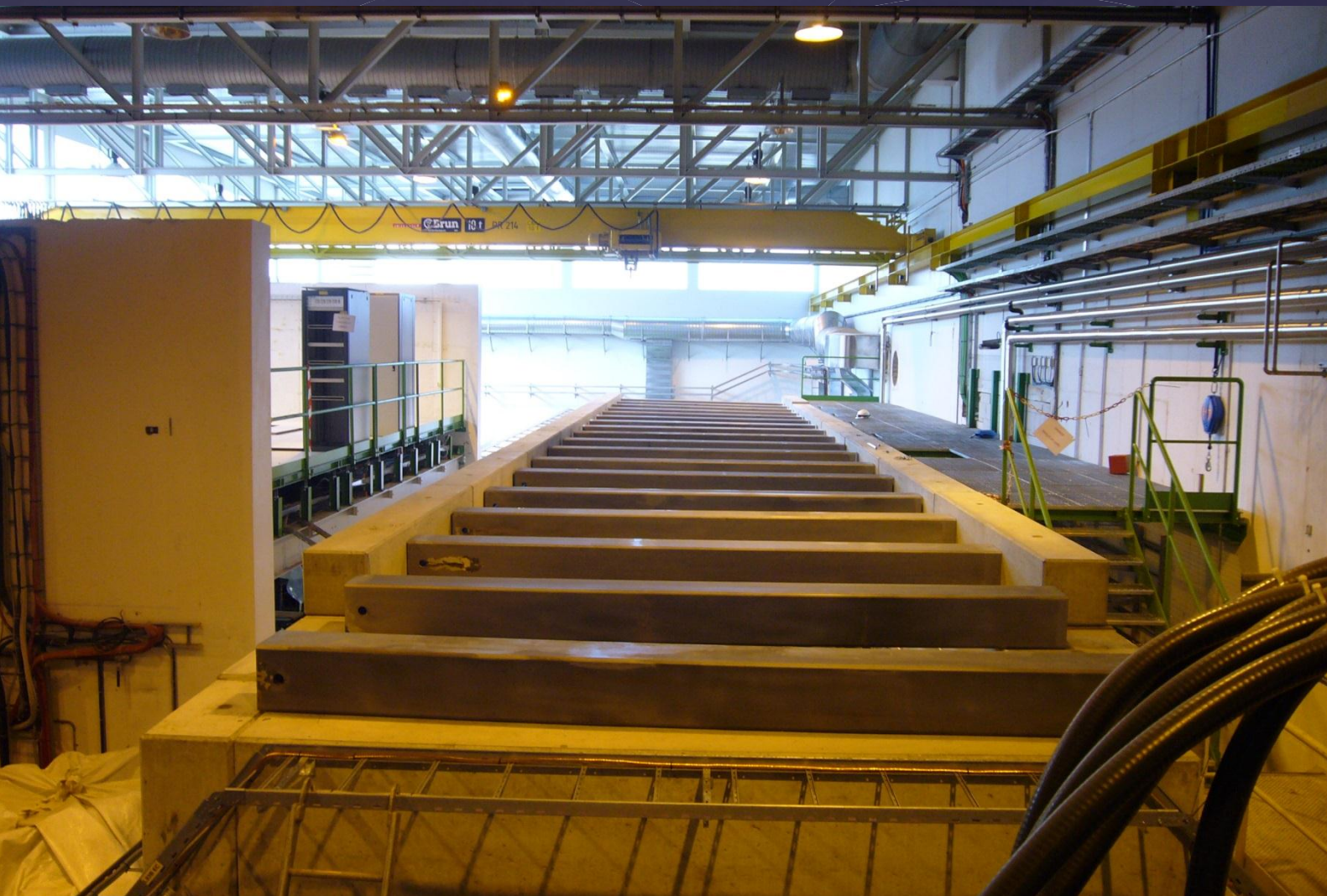
Linac shielding
