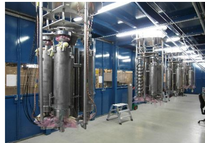
Cavity preparation area
