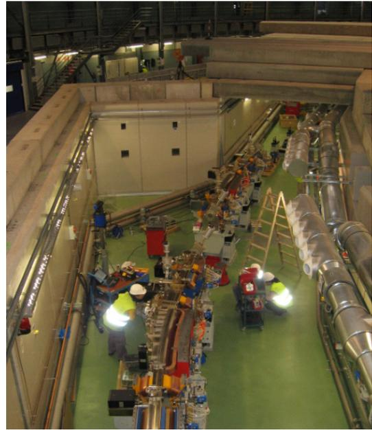
Figure 7: the sector placed in the girders with the magnets open.
