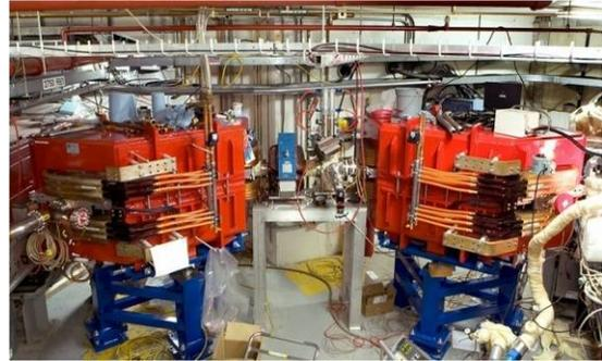
Figure 6: Dipoles installed in the Booster tunnel.
