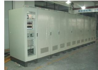
Figure14: The prototype pulse power supply for the injection bump magnet
