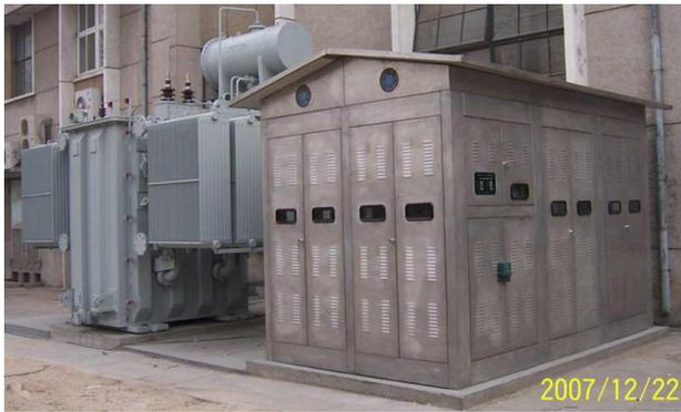
Figure 10: Choke and capacitor bank for White circuit of CSNS magnet power supply.
