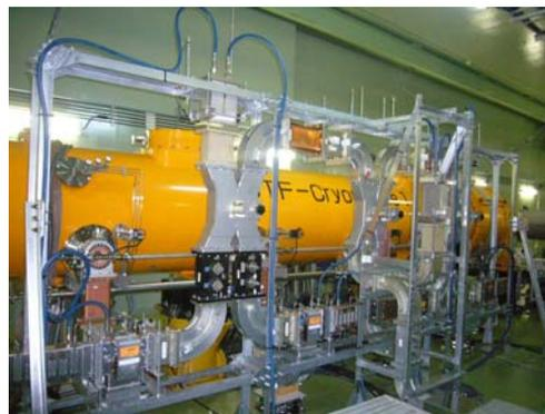
Figure 8: Installation of the cryomodule in the STF tunnel.
