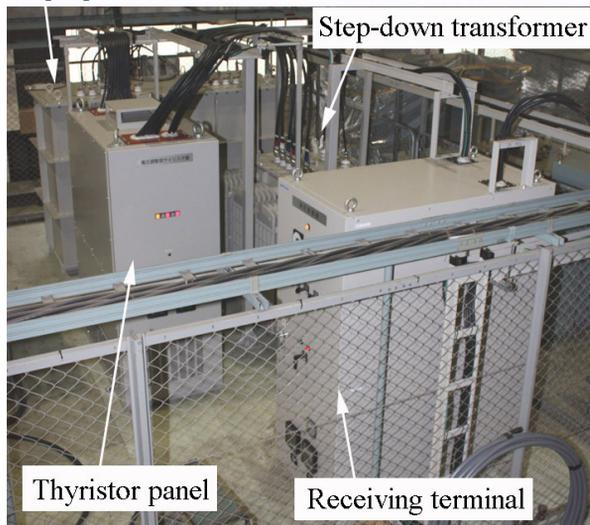
Figure 2: The main body of the new klystron power supply. A receiving terminal, a step-down transformer, a thyristor panel, and a step-up transformer with rectifier are shown.
