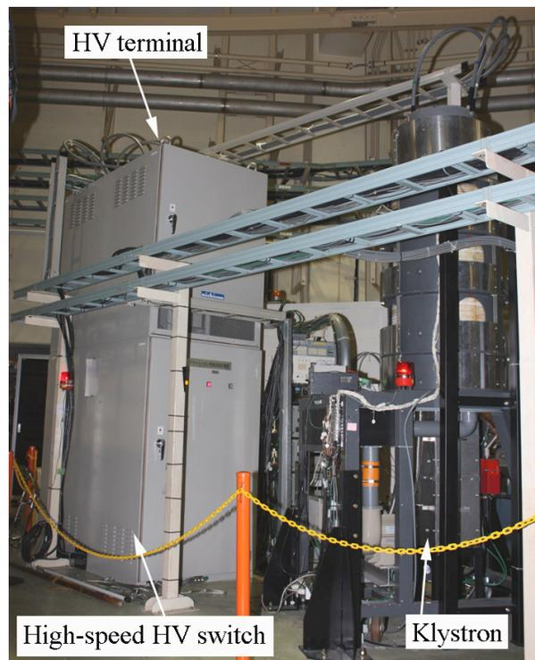
Figure 3: A high-speed HV switch and a HV terminal (left side) and the klystron (right side).
