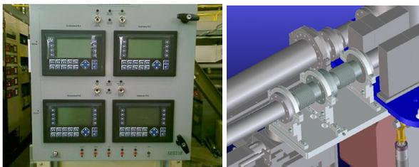
Figure 2: Left: Example of newly installed interlock system - PLC chassis, which are part of the beam current, lattice, and energy match interlocks. Right: Example of newly installed beamline aperture.
