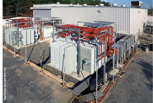
Figure 7: The New AGS MMPS Transformers.
