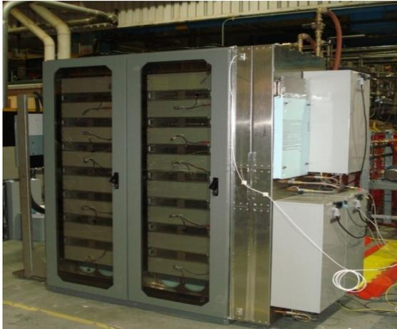
Figure 3: NSLS-II Power closed supply rack with air-cooling and air-to-chilled-water heat exchanger.
