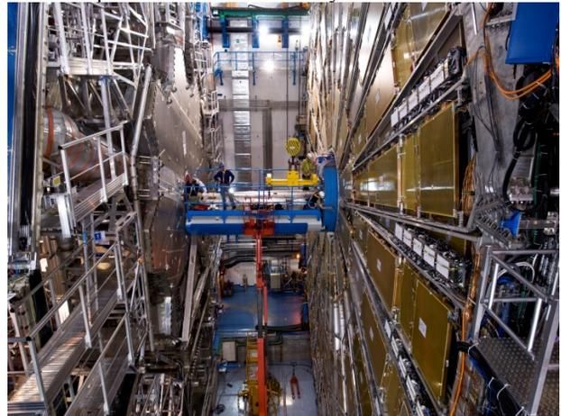
Figure 3: Installation of the last experimental beam pipe in the centre of the ATLAS detector.
