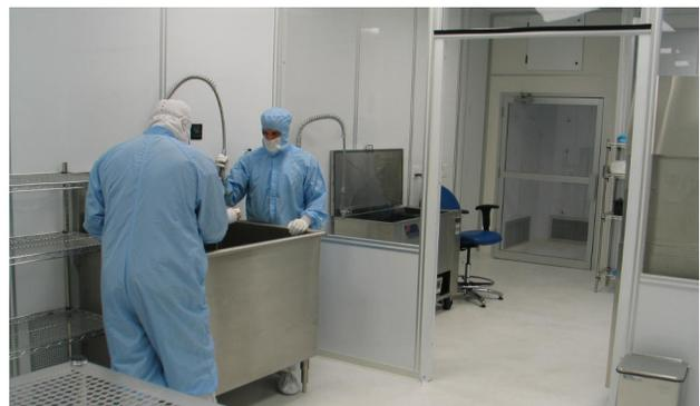
Figure 2: SLAC Coupler Cleanroom: the class 10 area is in the foreground and the class 100 area and air shower is in the background.
