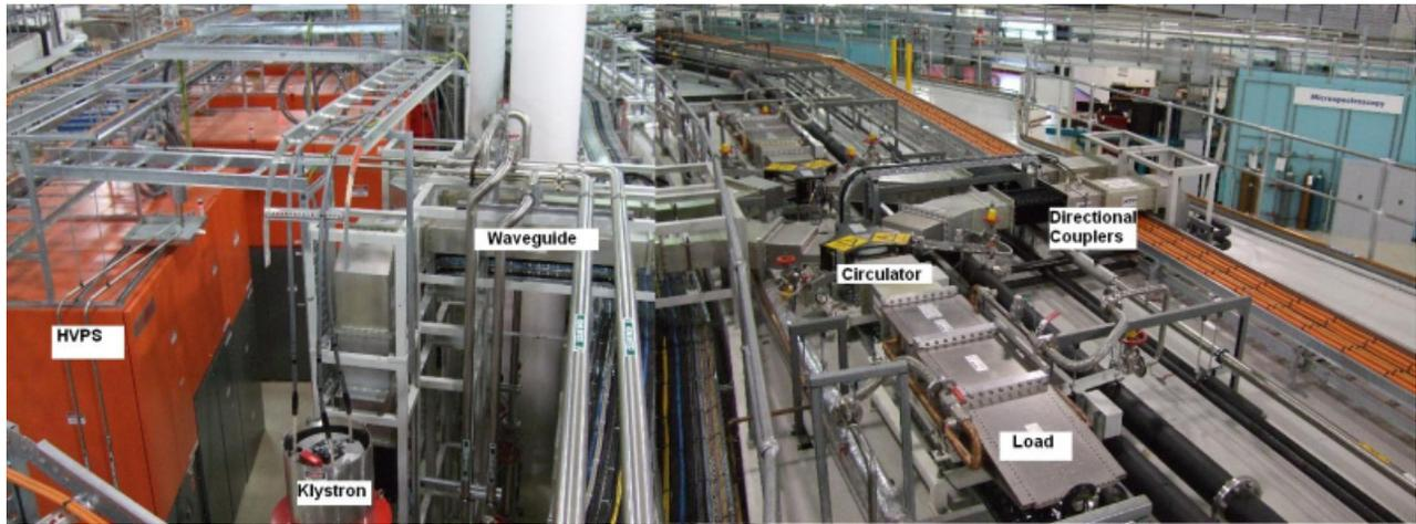
Figure 1: RF power distribution on Storage Ring tunnel roof for sector 7 RF.
