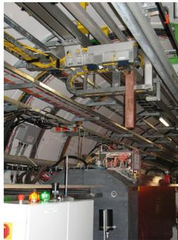
Figure 4: The remote handling system installed above the TANs in LSS1.
