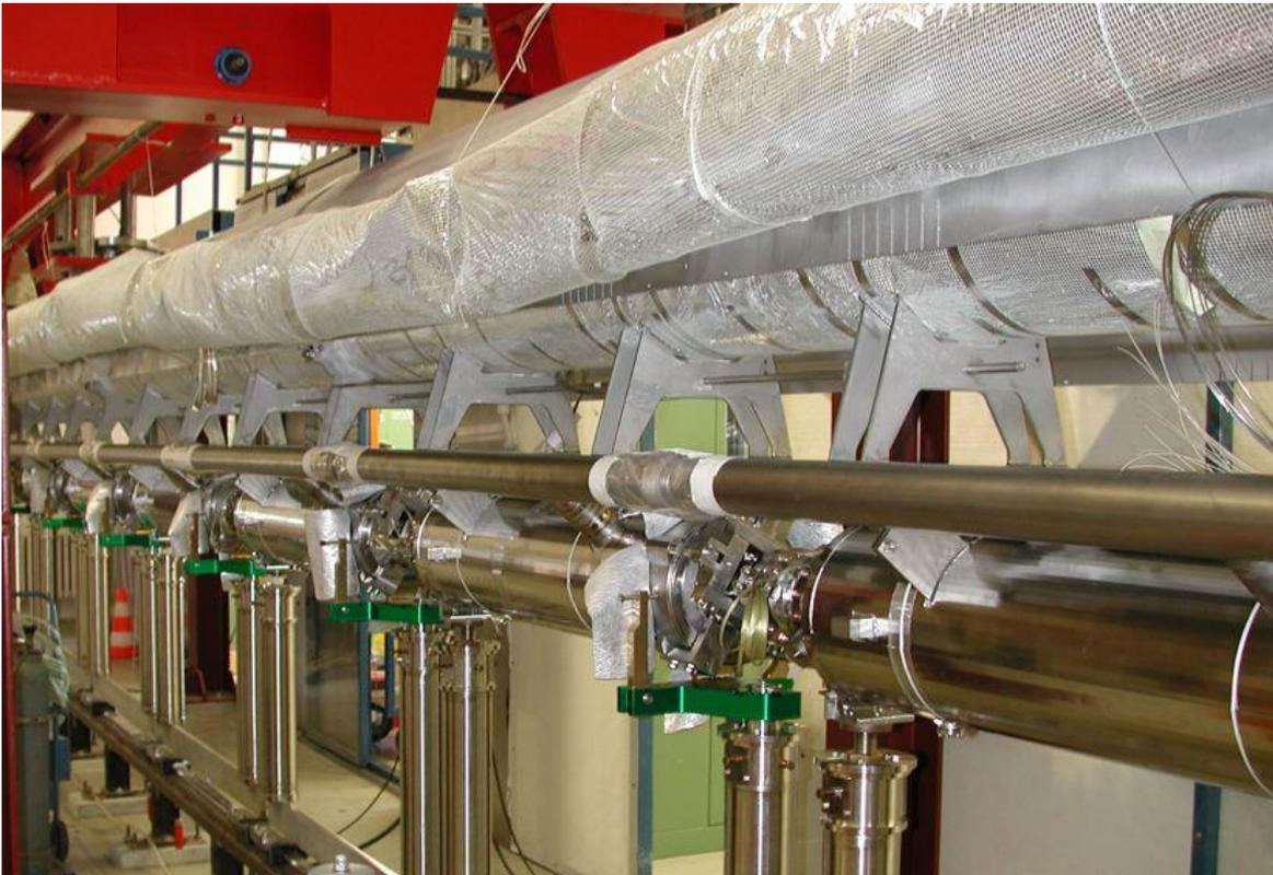
Cavity vessel and 2K helium supply pipe
