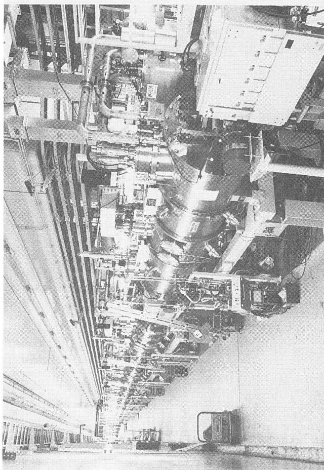
Fig.1 The string of cryostats for SC-RF cavities installed in the TRISTAN tunnel.
