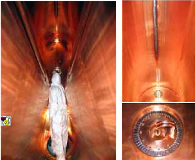
No major problems occurred during the power tests. Besides some harmless black deposits, an inspection of the cavity interior revealed no faults.
